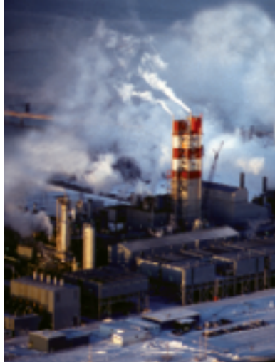
Figure 27 Operating an ammonia plant at relatively low temperature, high pressure, and low ammonia concentration maximizes the amount of ammonia produced.
