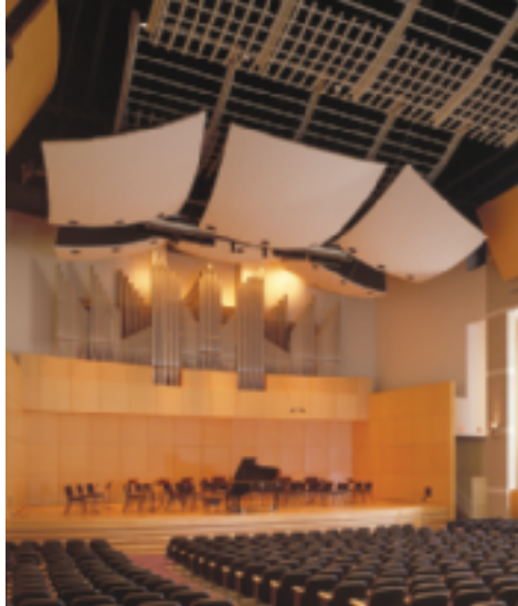
Figure 20 The Central Michigan University Music Building, like many concert halls, was designed by acoustic engineers. Sound-absorbing tiles (on the sides and rear) reduce unwanted reflections. The curved reflecting panels above the stage help gather and direct sound waves toward the audience.
